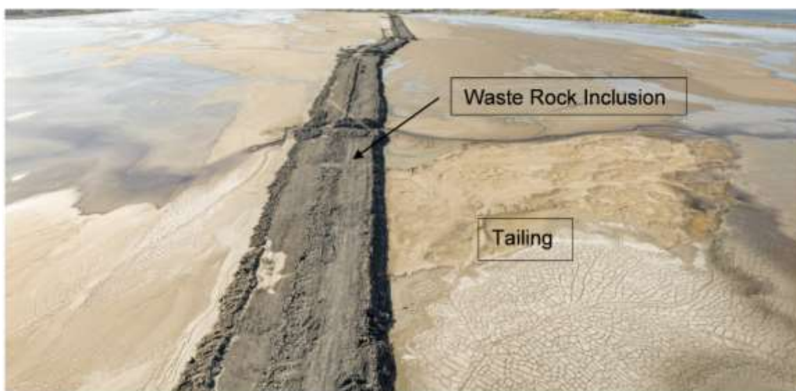
Figure 1.1: WRI in the Canadian Malartic mine tailings storage facility (photo taken September 2020)
