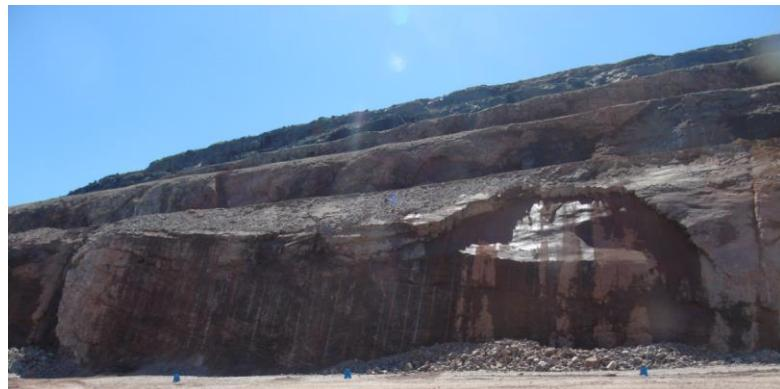
Figure 7.5 Slope failure and slabs observed on the southeast wall (bench 700-728)
