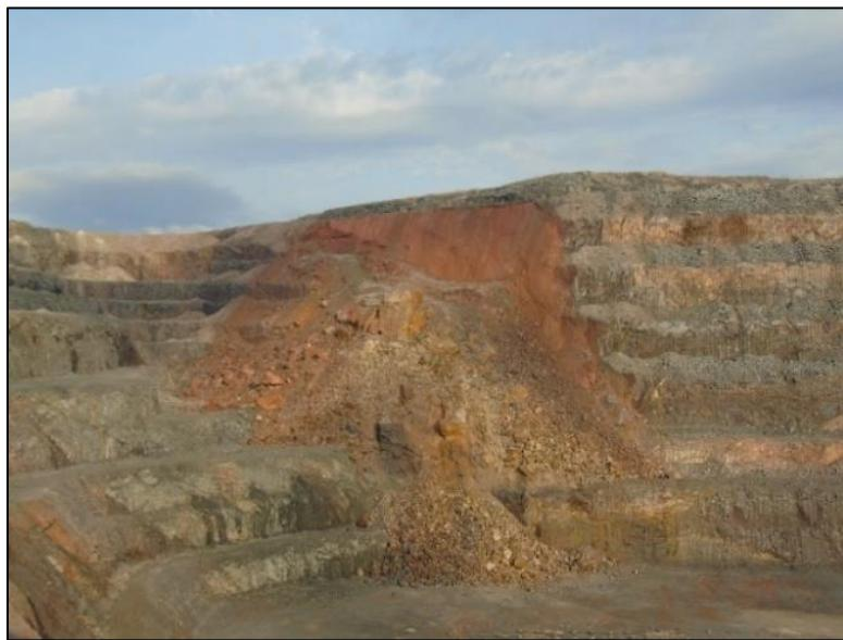
Figure 7.2 Southeast highwall post-failure photograph
