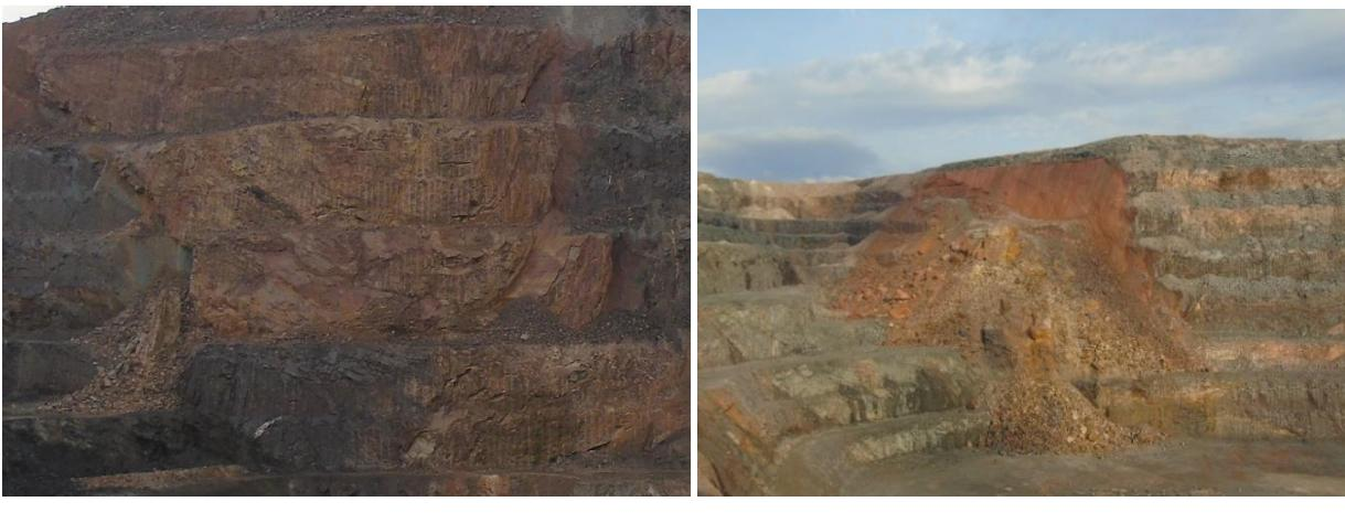
Figure 5.1 Southeast highwall: (a) Pre-failure (2018-07-02); (b) Post-Failure (2018-07-05)
