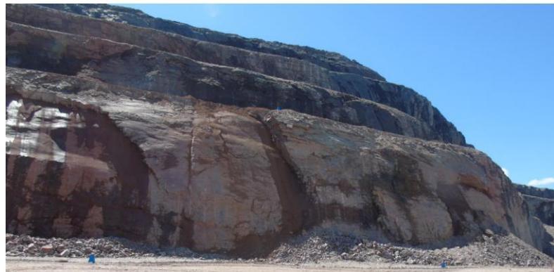
Figure 7.4 Slope failure and slabs observed on the southeast wall (bench 700-728)
