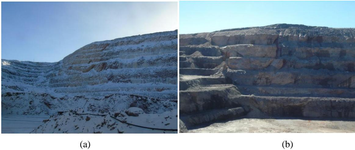
Figure 5.4 (a) Ice formation due to groundwater drainage surrounding the failure mass; (b) Post-thaw conditions of the slope surrounding the failure mass
