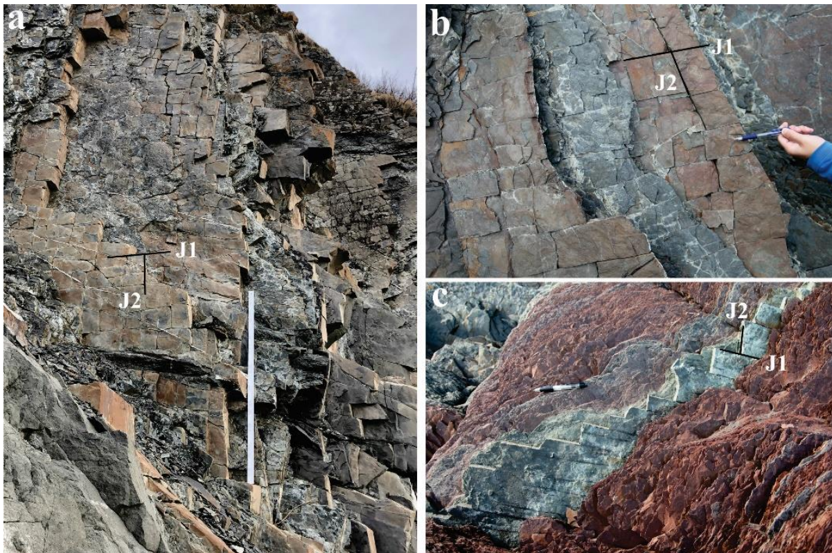
Figure 4.8 Ladder-pattern of orthogonal joints (sets J1 and J2) observed on sandstone bedding surfaces. J2 joints, which are less persistent than J1, extend across intervals between J1 joints and abut J1 joints at \sim 90^\circ angles. Scale in (a) is 1 m.
