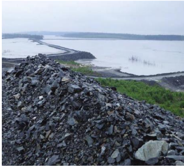
Figure 2.1 Waste rock inclusions in a tailings impoundment (taken from Bolduc & Aubertin (2014) with the permission of reproduction from Canadian Science Publishing)
